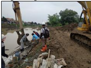
Gambar 22. Pengecoran capping beam
