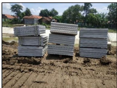
Gambar 4. Pengadaan material block lining
